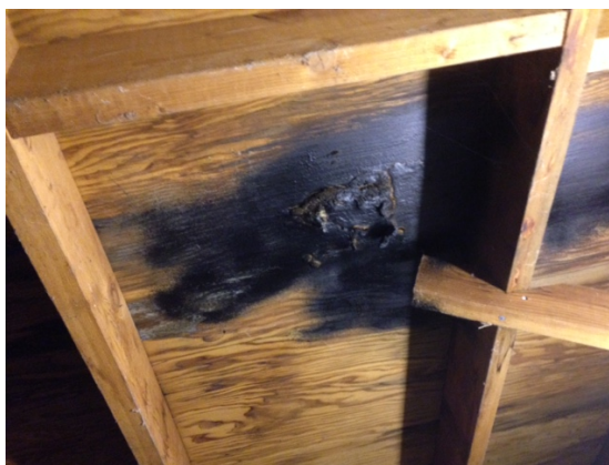
Observatory Roof Water Damage
